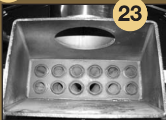
Last pass before exiting chimney
